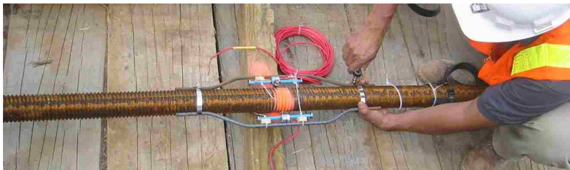
Figure 6.4. Photograph of VWSG Installed on Central Reinforcing Bar
