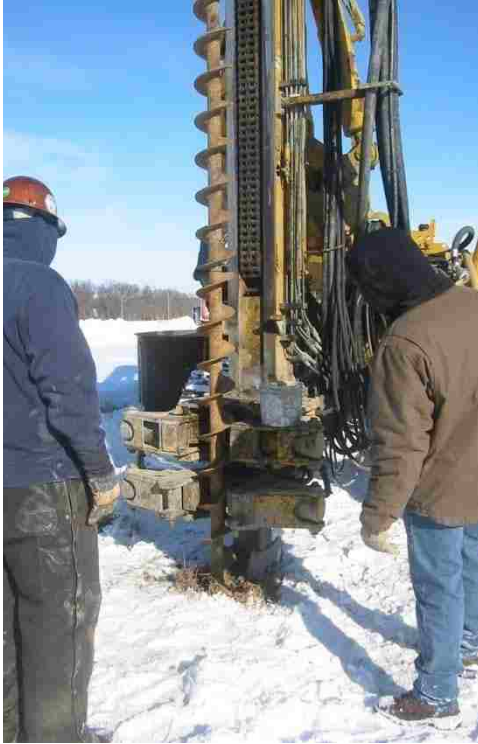
Figure 5.16. Micropile Drilling (Step 1)
