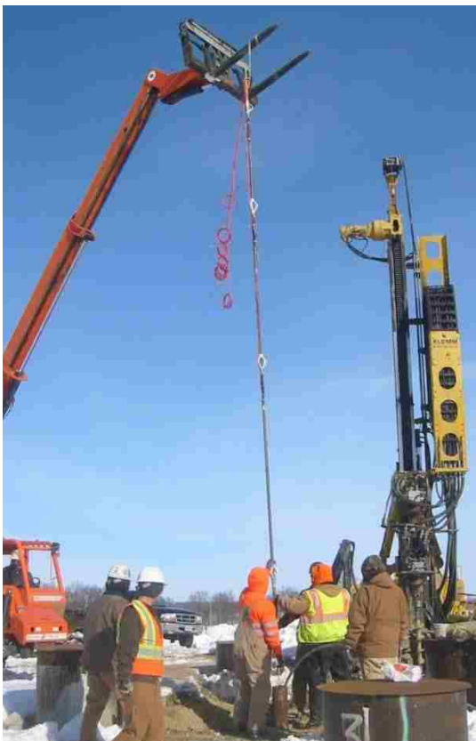
Figure 5.21. Placement of Central Reinforcing Bar (Step 7)
