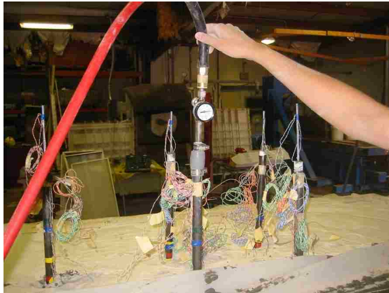
Figure 4.22. Photograph of Grout Pressurization and Casing Withdrawal (Step 5)
