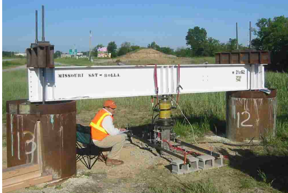
Figure 5.23. Axial Load Test
