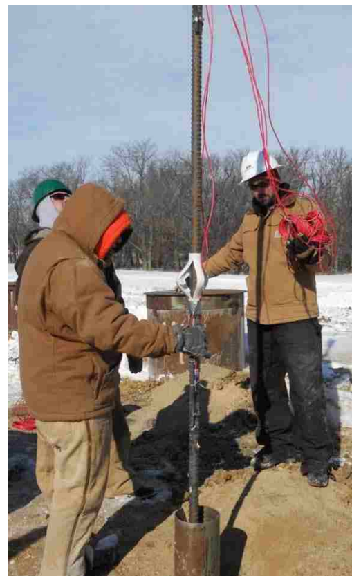
Figure 5.21. Placement of Central Reinforcing Bar (Step 7)
