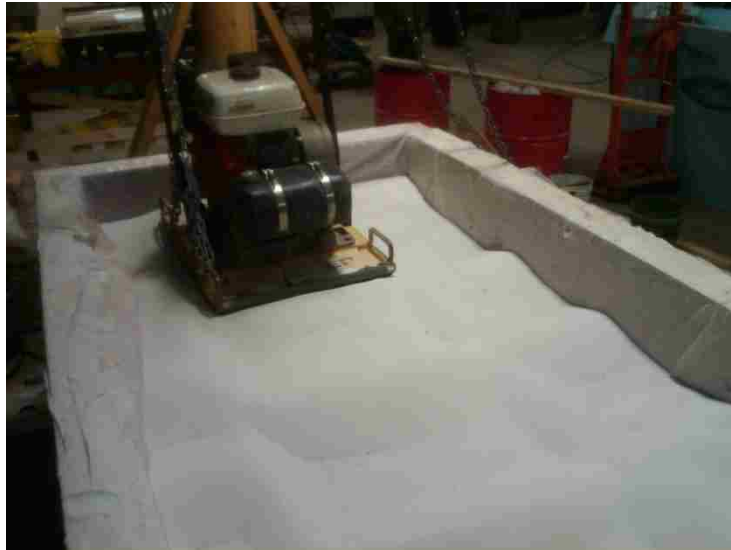
Figure 4.13. Photograph of Sand Placement using Vibratory Compactor
