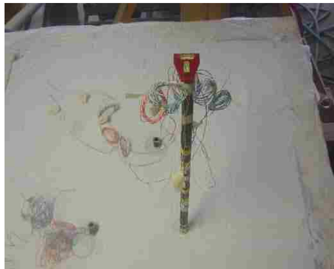
Figure 4.20. Photograph of Casing Installation (Step 2)
