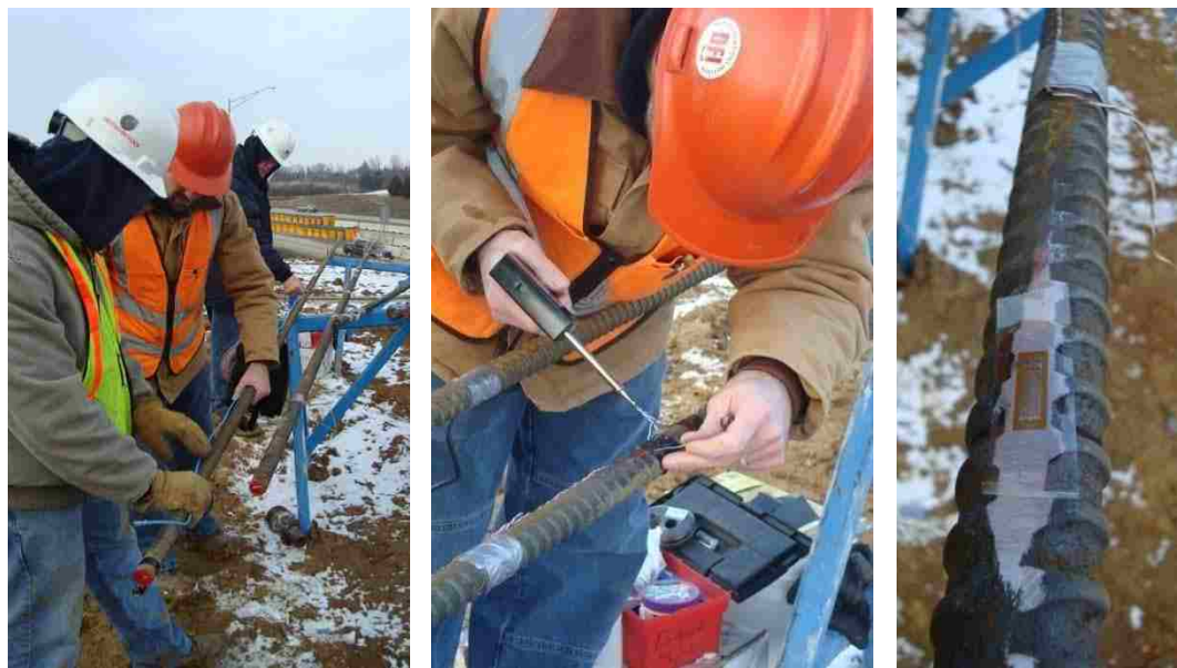
Figure 3.10. Photographs of Strain Gage Installation
