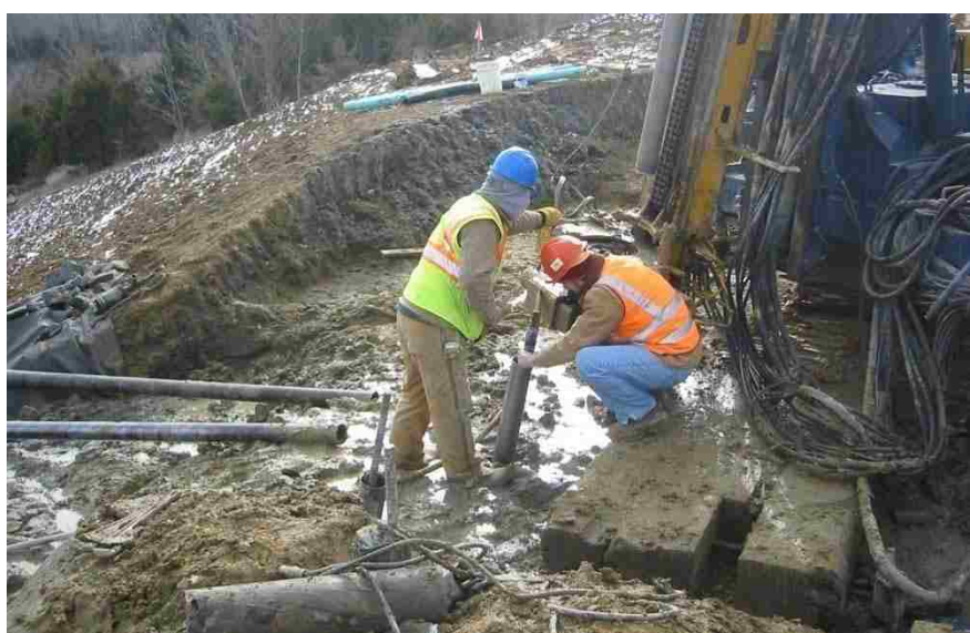
Figure 3.9. Photographs of Completed Micropile 58-G
