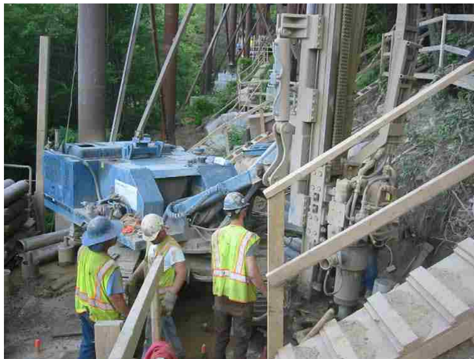
Figure 6.6. Photograph of Micropile Drilling (Steps 1 and 2)
