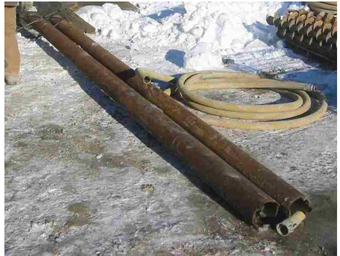
Figure 5.17. Micropile Casing (Steps 2 and 3)
