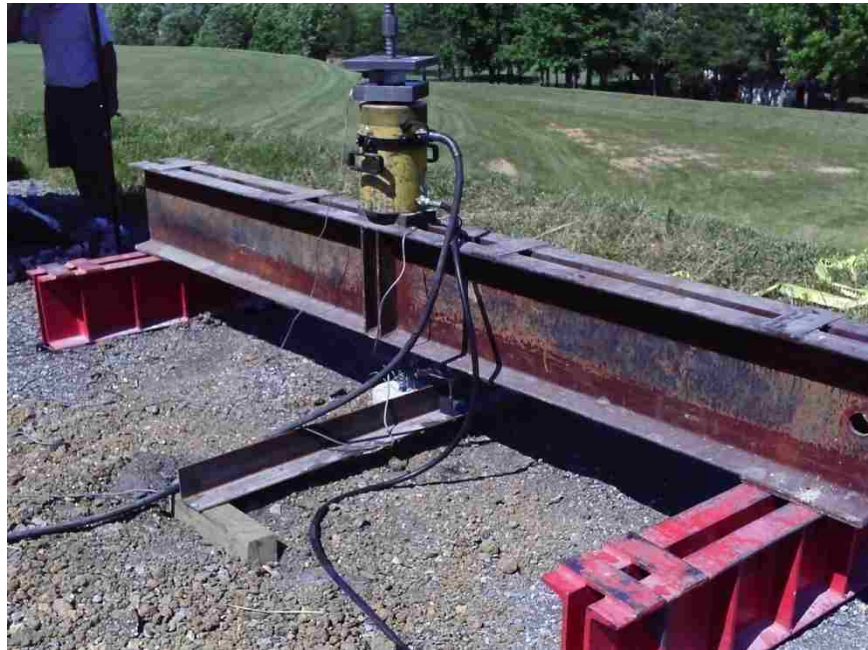
Figure 3.4. Ber Juan Load Test Setup
