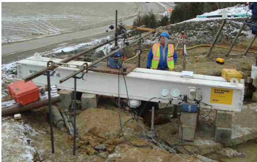
Figure 3.11. Photograph of Colt RR Proof Load Test Setup
