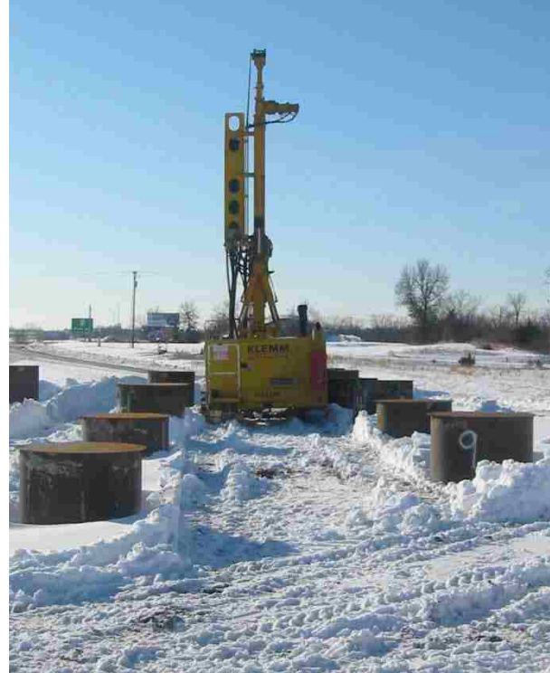
Figure 5.16. Micropile Drilling (Step 1)
