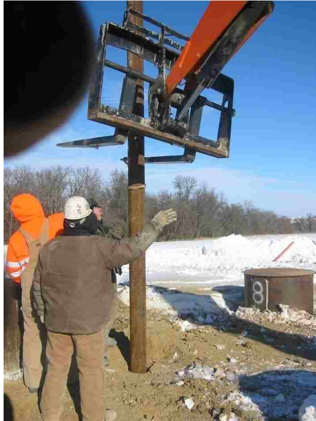
Figure 5.18. Installation of Micropile Casing (Step 4)
